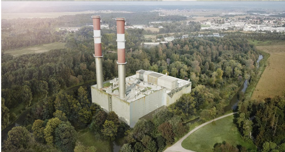
"Reclaiming Abundance" (Mellach gas and thermal power plant), Digital print on dibond behind acrylic glass, 100 x 52,7 cm, 2021
